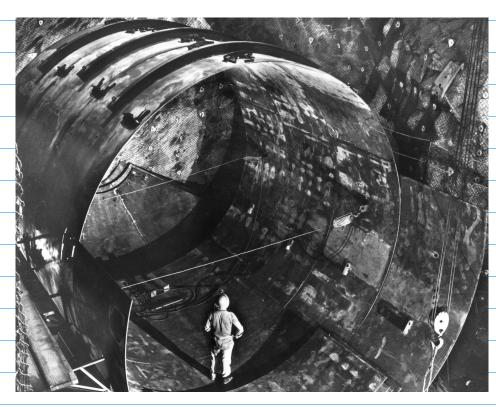
TANK FILLED WITH 380,000 LITERS OF DRY CLEANING FLUID C2 Cl4.
